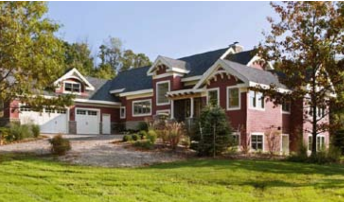
Burnside's Inn (residence), Dexter, MI 4,010 sq. ft. 0.86 ACH50 HERS Index of 37 (includes solar)
