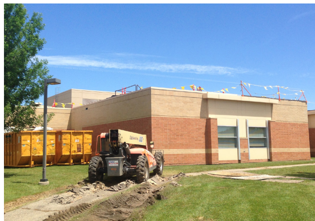
Figure 2. Roof replacement in progress
