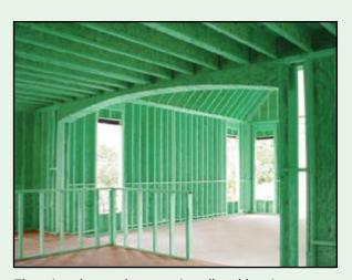
There is only one chance to install mold-resistant wood: when the home is built. The FrameGuard® treatment prevents mold growth and thus reduces airborne mold spores.
